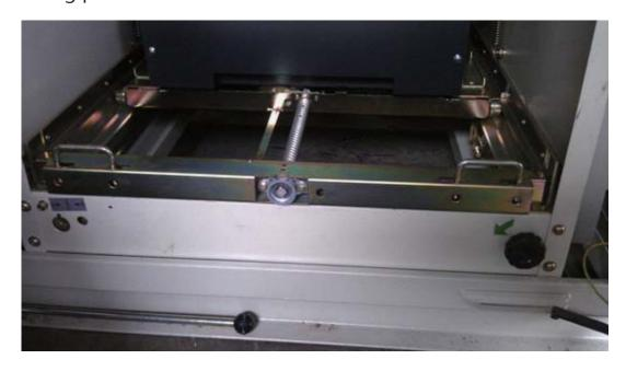
1. Withdraw the VCB from SERVICE position to TEST position.
