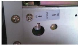
3. To close the ES: Insert the operation lever into the hole, and then turn counter clockwisely until the lever is in vertical position.
