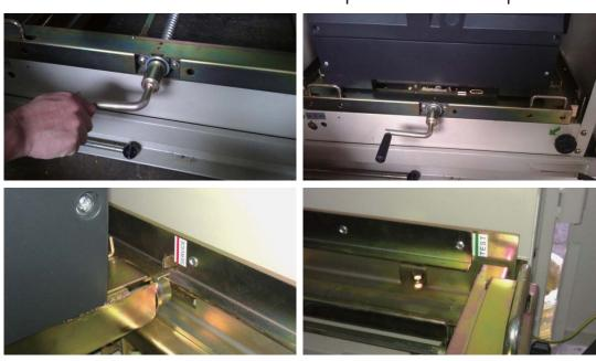
2. Turn the switch counter clockwisely to release the interlock.
